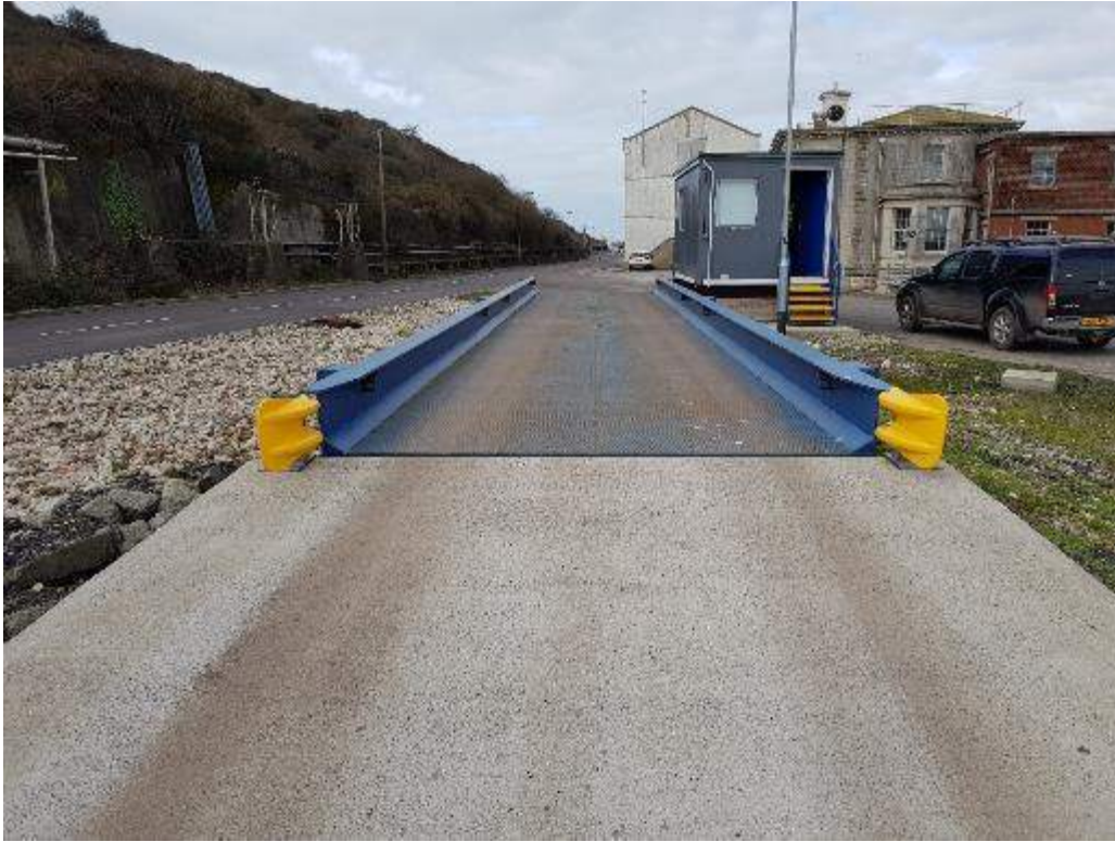
Photograph 5: Weighbridge , northwest corner of site
