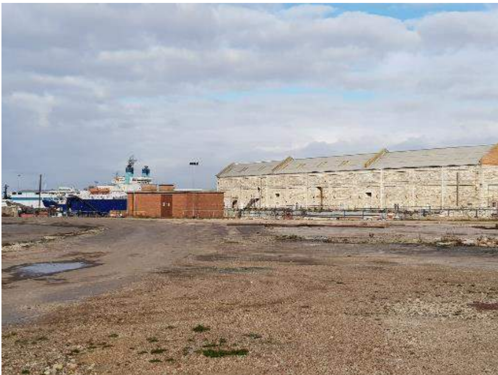
Photograph 4: Electricity substation adjacent to northern site boundary
