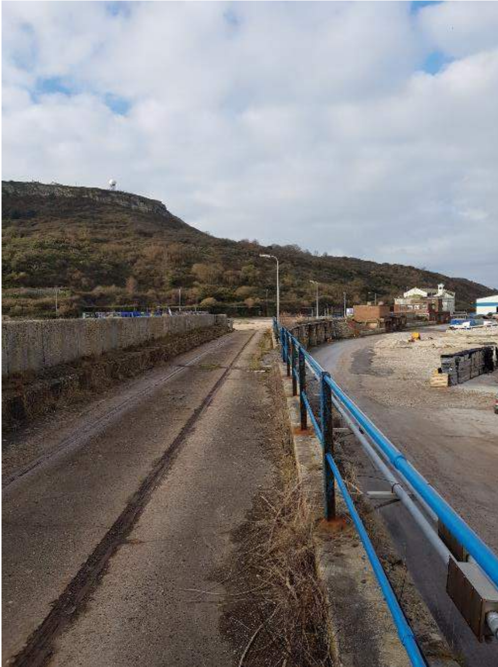
Photograph 9: Retaining structure along northern site boundary
