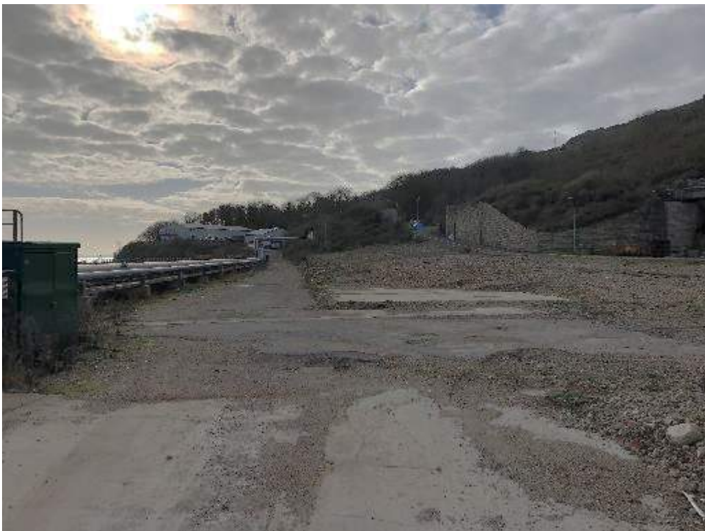
Photograph 6: Above ground pipeline along eastern site boundary
