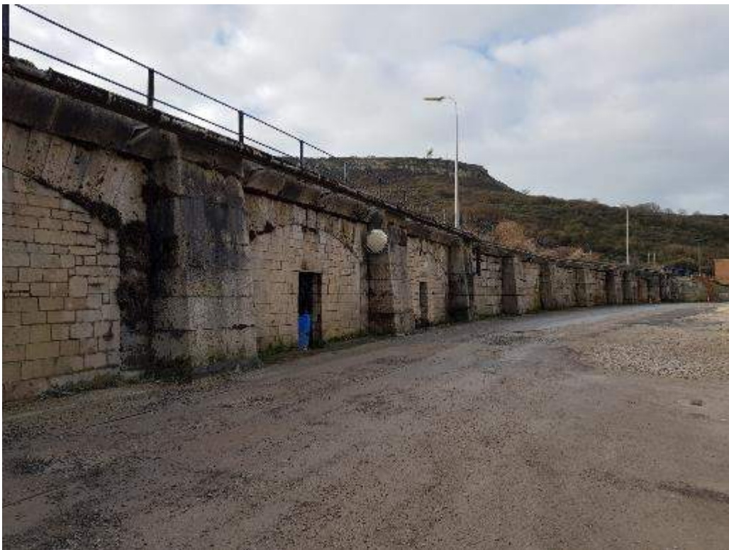
Photograph 8: Retaining structure along northern site boundary
